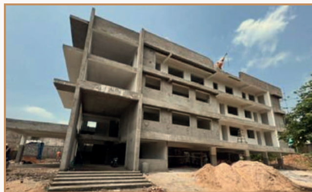
Construction Progress: A Modern Research Facility Takes Shape
